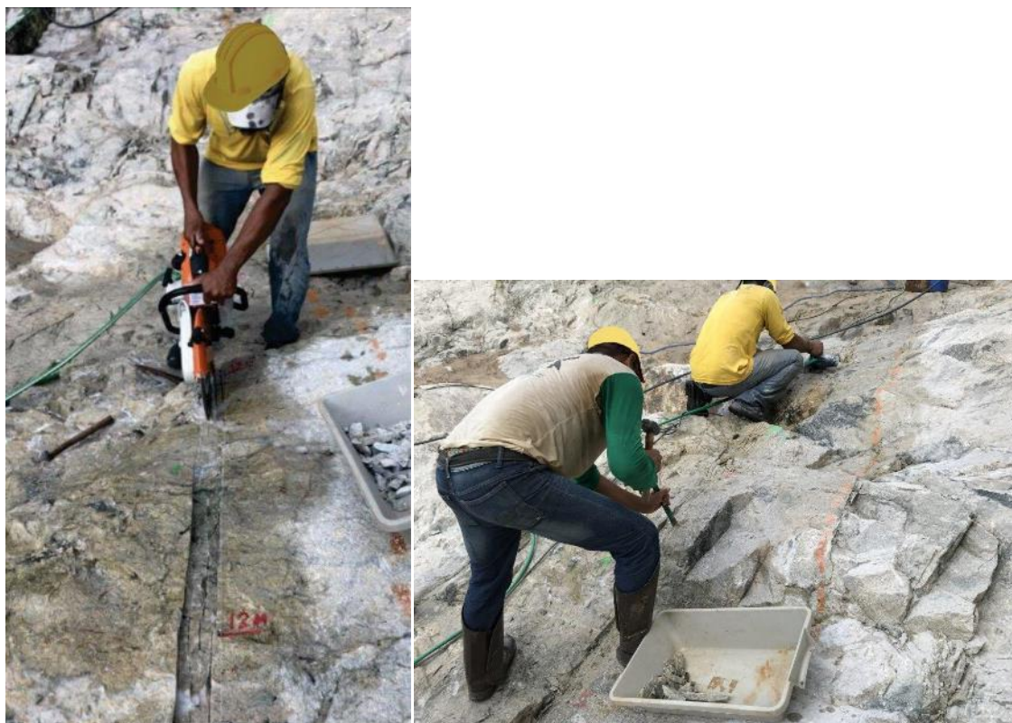
Figure 9.15 PNP Channel Samples Collected in Hard Rock Using Electric Saw with Diamond Blade
